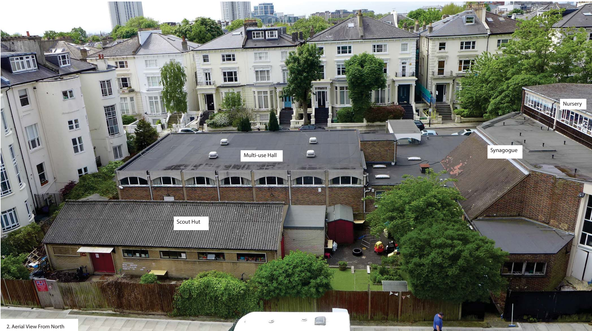
2. Aerial View From North
